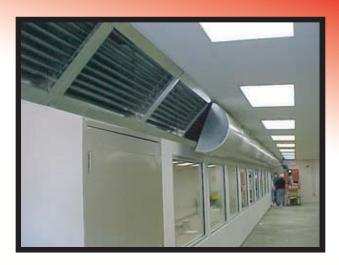
**Laminaire** TM Radial Air Diffuser by Patriot Range Technologies LLC The latest design in the Radial diffuser system provides for a 45-degree angular mixing box. This revolutionary design provides the best "on-range" airflow performance in the industry and is the basis of the newest military airflow performance criteria under the MIL/HDBK 1027-3B-15C.
